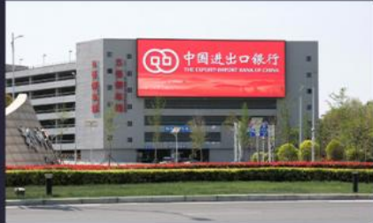
Wall mounted installed on the Airport Hotel Building
