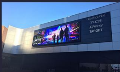
Embedded Installation in the Building
