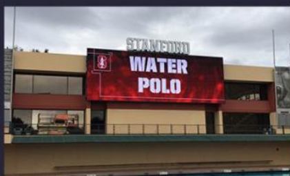
Installed by the Swimming Pool
