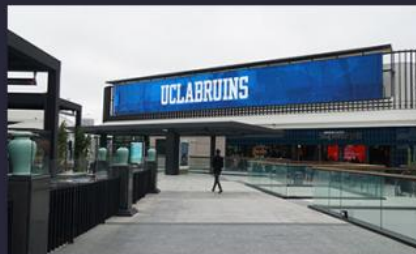
Shopping Mall Entrance steel structure stacking installation
